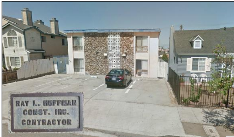
Figure 2.7 “Six Pack” Apartment Building in San Diego
